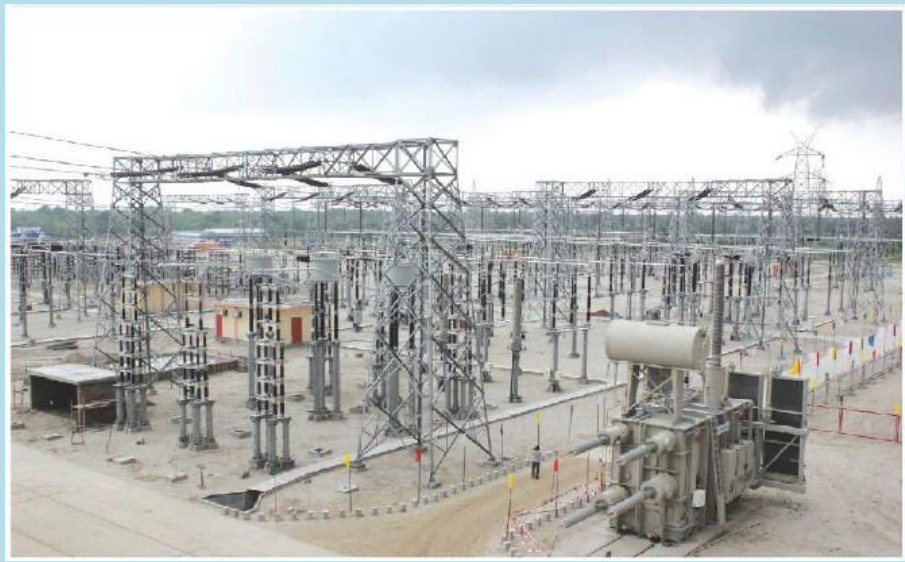
Figure 21: Bangladesh India Power Transmission Plant, Bheramara (Kustia)
