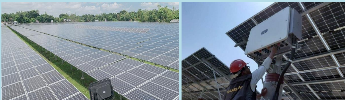
Figure 24: Bangladesh's Largest (73 MW) Solar Power Plant, Mymensingh
