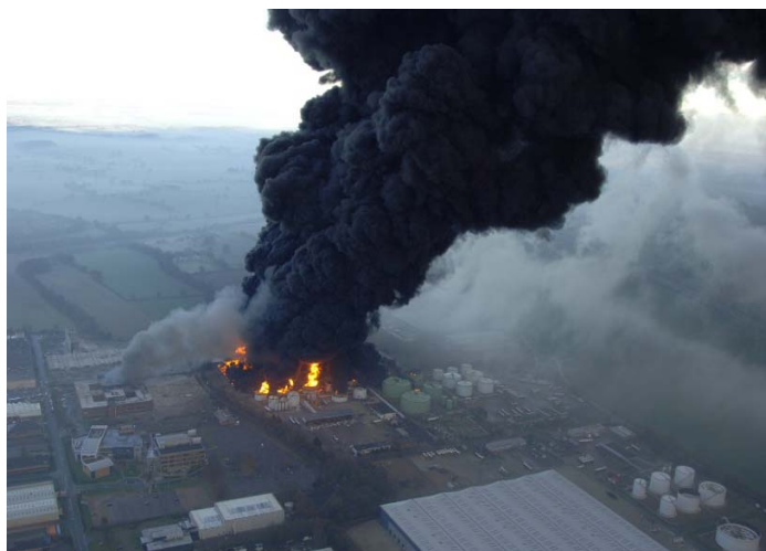
Group of tanks on fire with secondary fire in the neighbourhood
