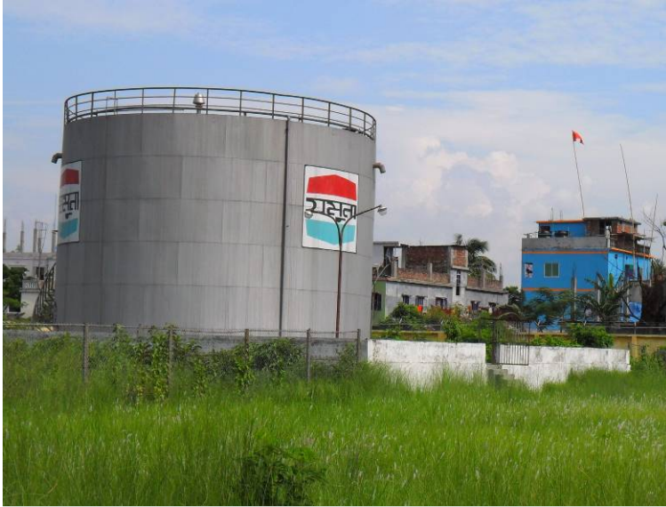
Storage tank at depot with „access gap“ in bunding
