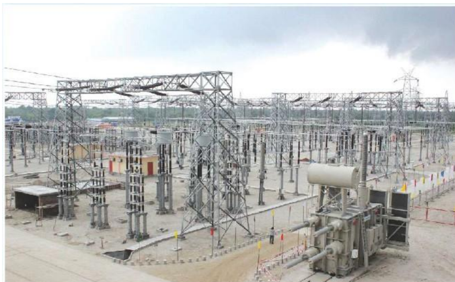
Figure 20: Bangladesh India Power Transmission Plant, Bheramara (Kustia)
