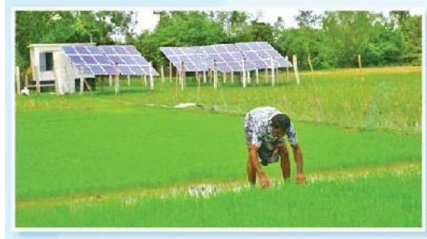
Figure 25: Solar Pump System in Rangpur District
